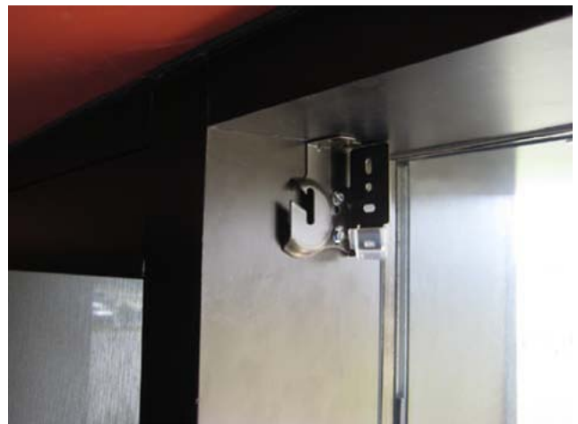
• Side mount application shown. As shown can be mounted top, side, or back mount, as well.
